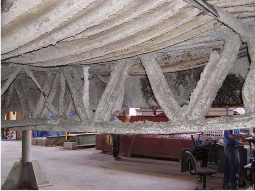
Figure 2. Buckled truss webs and bowed metal deck
